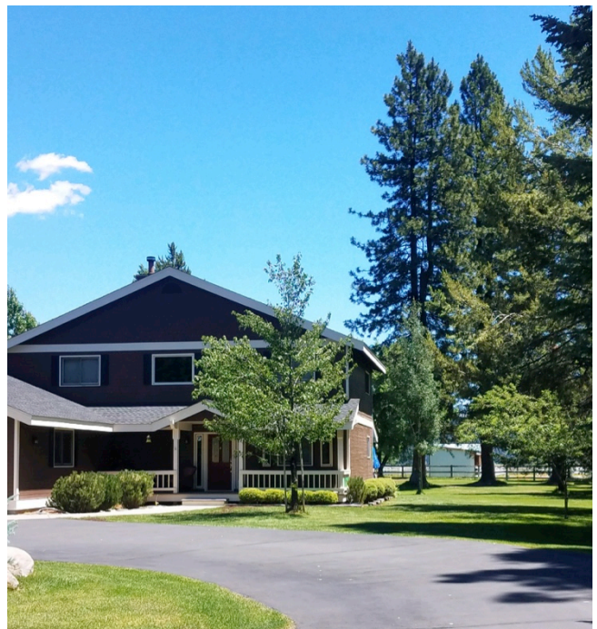
Figure 11: This home has no ladder fuels and is kept very green with a circular driveway for emergency equipment access
