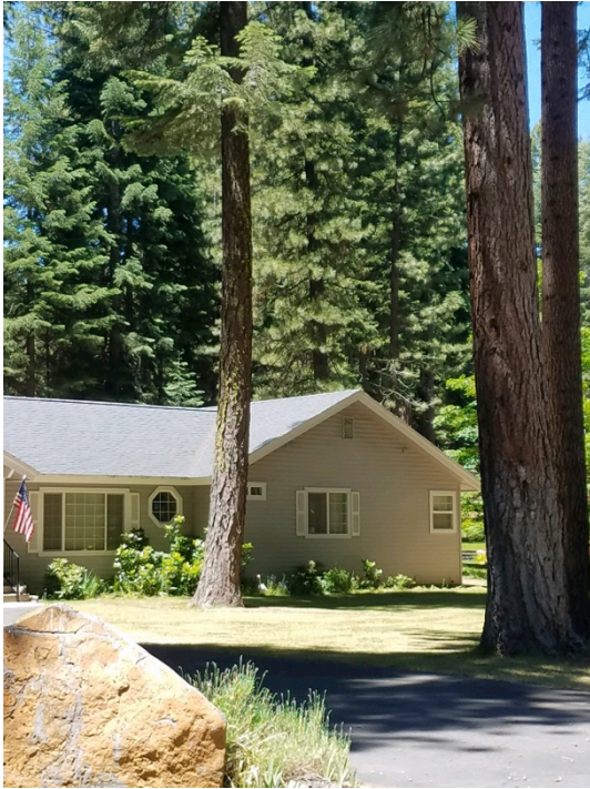
Figure 8: Trees are limbed high and green vegetation will reduce the spread of fire to and from the structure
