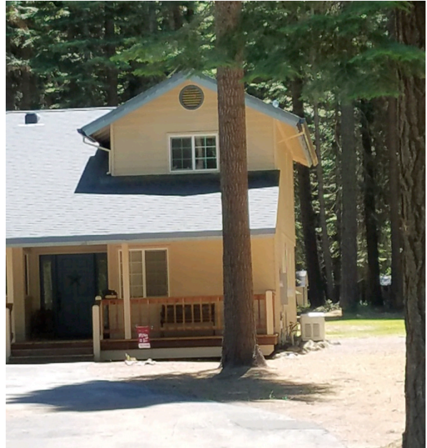
Figure 9: This home has trees limbed up and a clear area around the structure. Under the deck is maintained free of dead materials.
